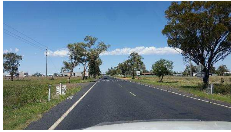
Inner edge / 60km/hour sign (landscape opportunity both sides) NEVERTIRE-BOGAN RD SOUTHERN APPROACH (FROM TOTTENHAM)
