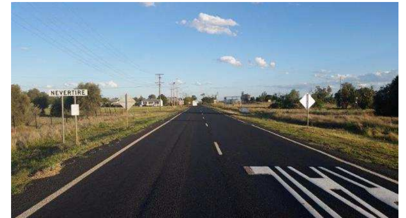
'Nevertire' black on white village sign (retain but add Key Facilities Sign)
