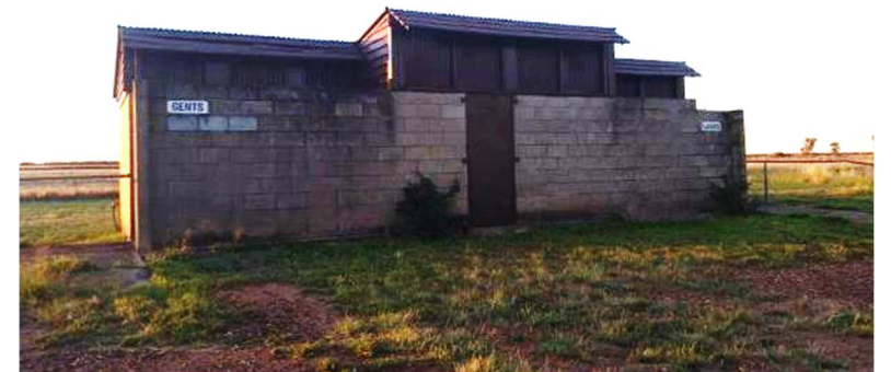
Discuss upgrades required to toilet block (especially if camping allowed)
