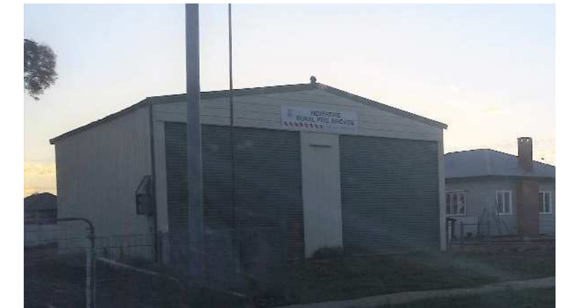
Rural Fire Service Shed – Narromine St
