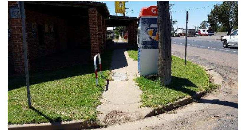
Clyde St (widen footpath / add kerb ramps as part of new blisters)
