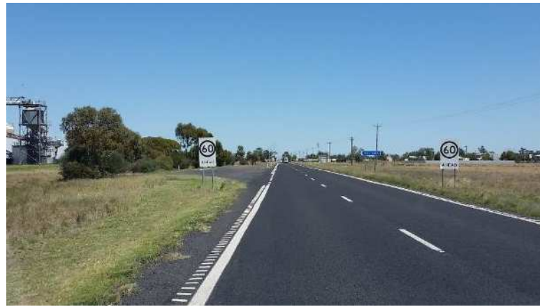
60km/hour ahead speed signs and outer Rest Area (add landscape)
