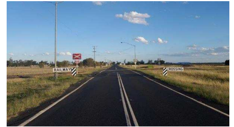
Rail crossing is quasi-western gateway (may need upgrading in future)
