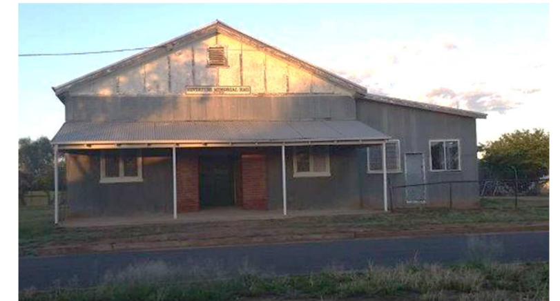
CWA Hall (repair/repaint/clean entrance/new path/open up to park)
