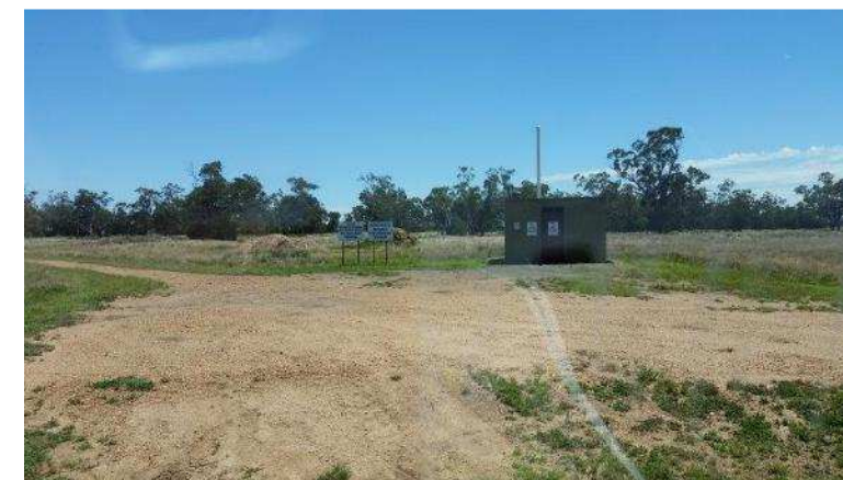
Sewage Treatment Plant (possible future re-use of treated water)
